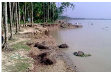
Fig. 2. Affected area by flood
